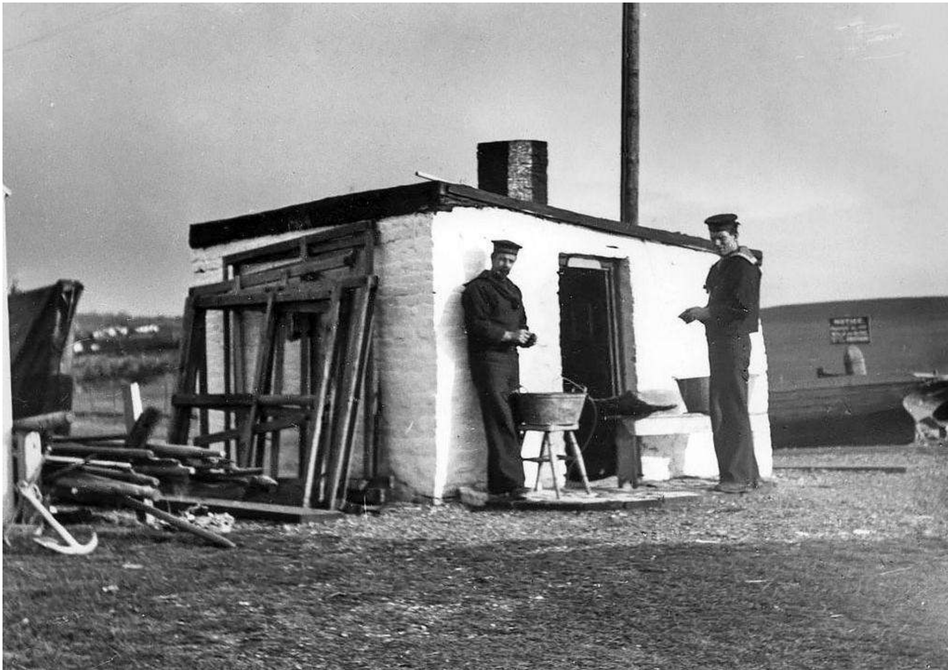
#6: Martello Tower #50 (used to build coastguard station), 1896
